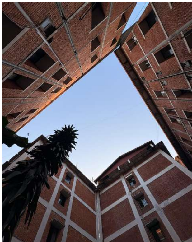
Figure 2: Multi-storey wing of the hospital complex
